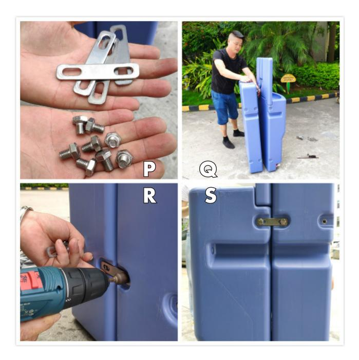
6. Using four screws, attach fresh water tank to the waste tank. To do this, line up bracket slots, then insert screws into pre-drilled holes. Using a drill, tighten to secure.
